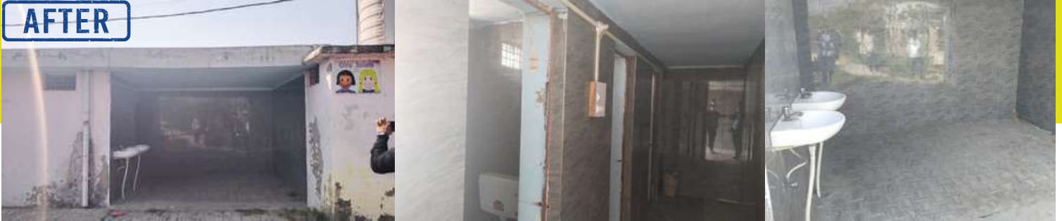
In picture - Before & after Re-construction of the Garhi Bohar school washroom.
